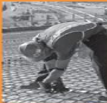
TYING REBAR BY HAND
